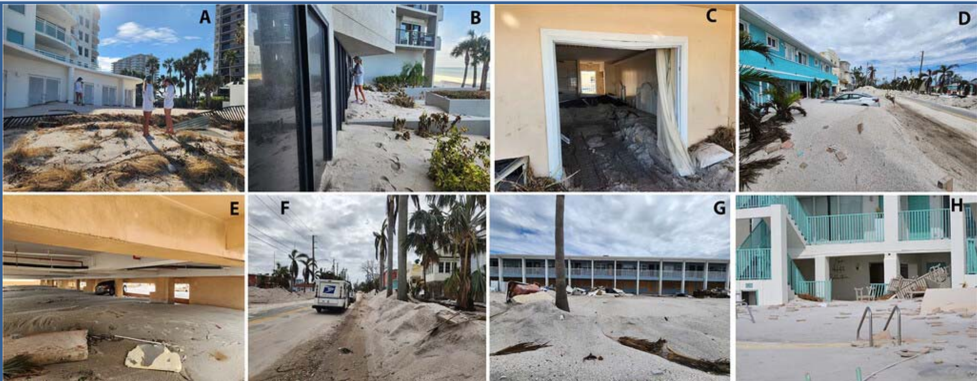
Figure 7. Sand overwashed into beach-front infrastructures. (A) Sand deposited outside a storage unit, north Sand Key; (B) sand deposited outside a hurricane glass door, north Sand Key; (C) sand deposited inside a beach-front house, north Sand Key; (D) sand was overwashed around and through beach-front buildings and deposited along a coastal road, Treasure Island; (E) sand deposited within a parking garage, south Sand Key; (F) up to 1-m-thick sand deposited along a coastal road, Treasure Island; (G) sand deposited in a hotel parking lot on the landward side of a coastal road, Treasure Island; (H) sand filled a swimming pool, south Sand Key.
